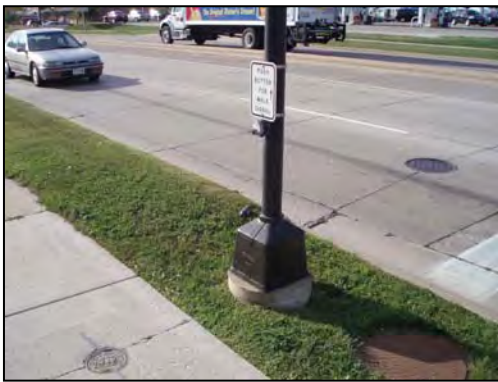
Button that can be reached from the sidewalk.
