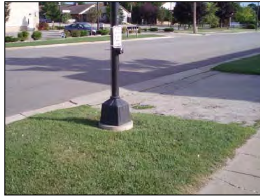
Button that cannot be reached from the sidewalk.
