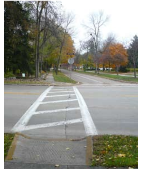
Crossing at Broadway and Ridgeway Boulevard
